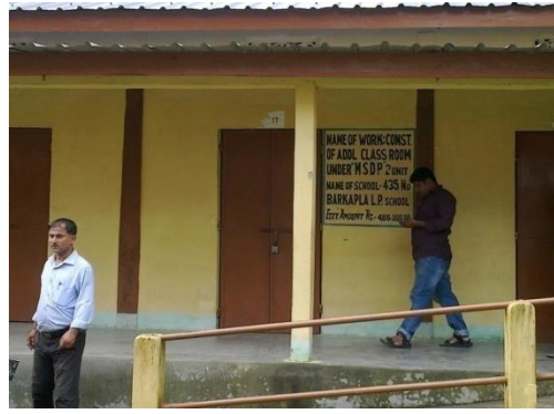
School Additional Class Room under MS DP
