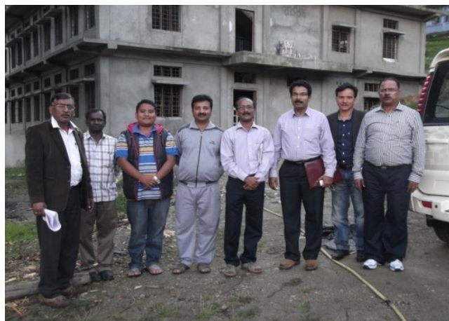
Girls' Hostel under Construction- Vivekananda Kendra Vidyalaya – Shergaon GP Kalaktang Block
