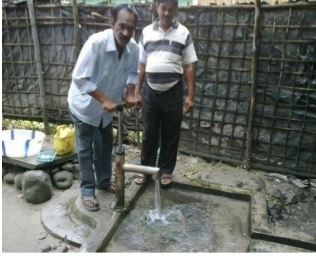
Drinking Water Scheme
